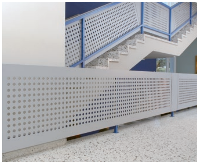
STAIR RAILING - HOLE MILLING
