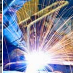
Industrial Metal Works
