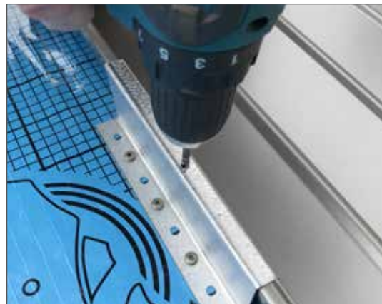
2. Drill a hole perpendicularly at the top of the turned directional clip
