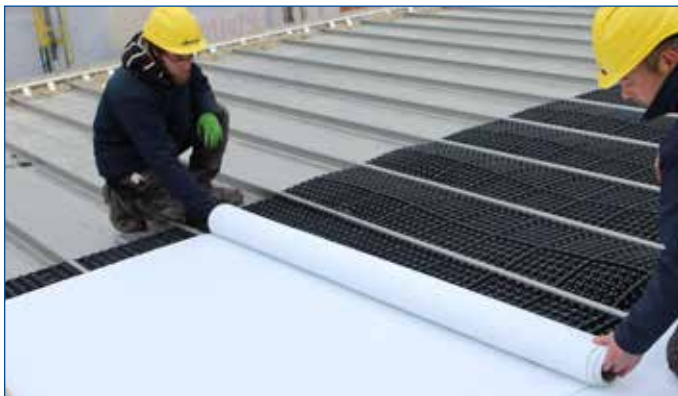
Roll out a fleece layer over the Urbanscape drainage and storage layer.
