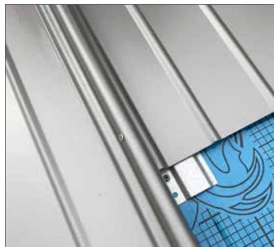
4. Finally, swivel in the next profiled sheet
