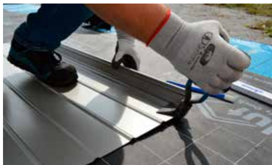
3. Position the curved folding pliers on the left and set up the bottom boom slightly again.
