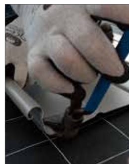
2. Position the curved folding pliers on the right and set up the bottom boom slightly.
