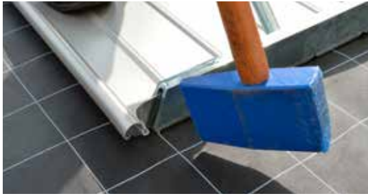
5. Knock with plastic hammer during installation.
