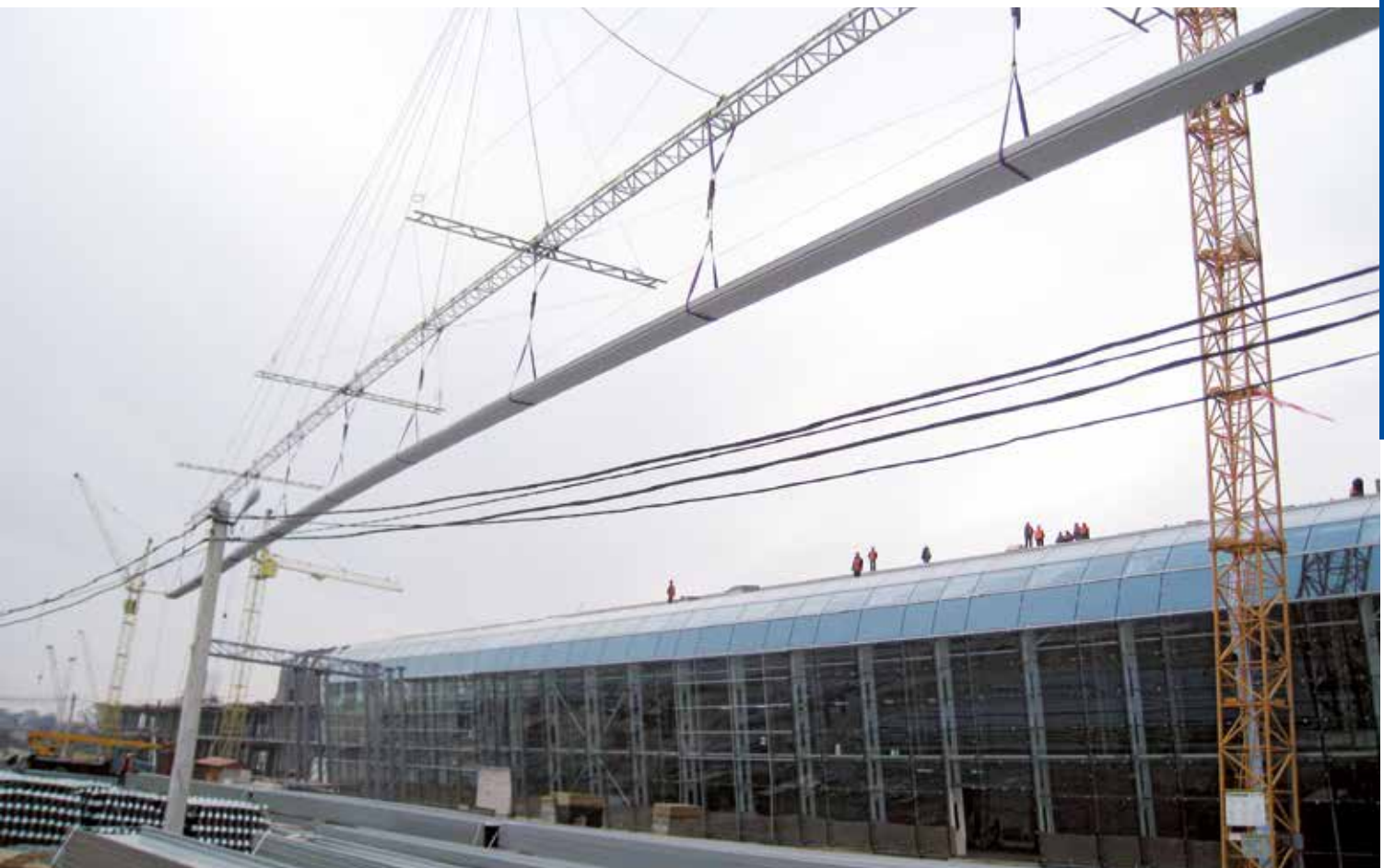
Special spreader beam for extra long profiled sheets.
