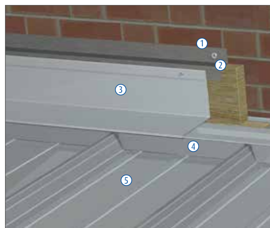
Wall connection at ridge
