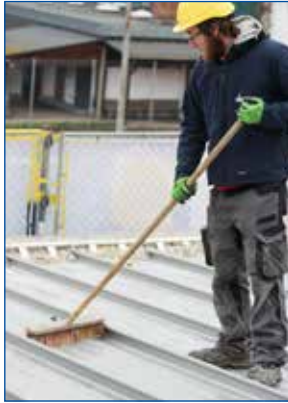
Sweep a RIB-ROOF roof.
