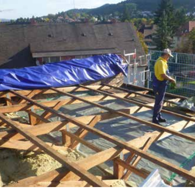
The use of wooden substructures saves weight and is, therefore, often the only appropriate solution in the case of renovation.
