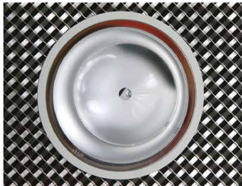
Fitting of lights, Mesh: Atlantic (4)
