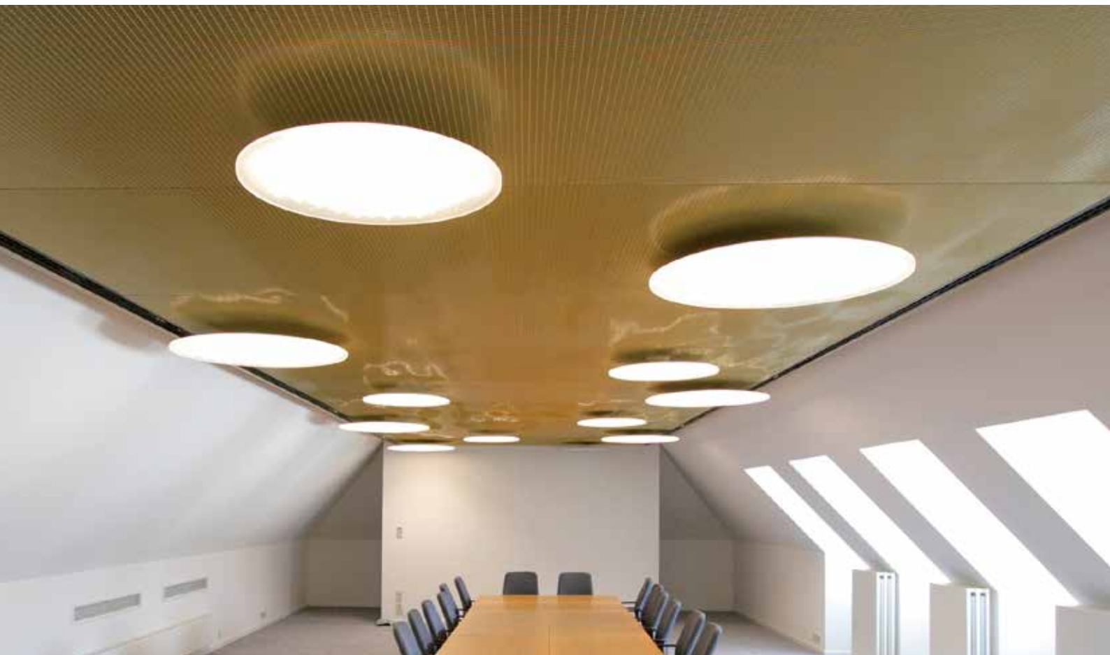
„König von England“ (King of England) Ministry Building, Stuttgart, Germany. Architect: zsp architekten. Mesh: CMP Alu 6010 (7)
