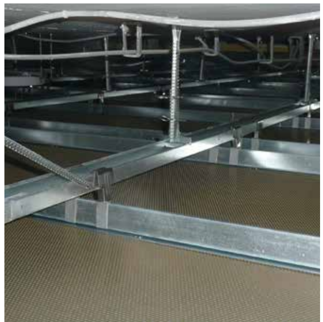
Trouble-free connection to adjoining components (9)
