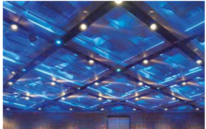
Tonhalle, Dusseldorf, Germany. Architect: HPP Hentrich-Petschnigg & Partner. Mesh: Omega 1540 Bronze (special mesh) (10)
