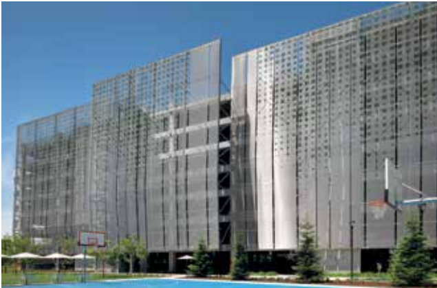
SAMSUNG PARKING GARAGE, SAN JOSE, USA
