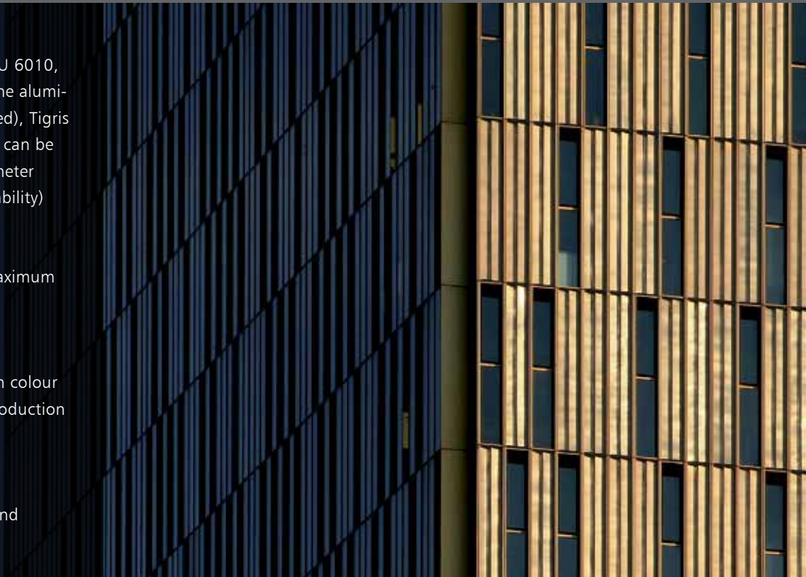
Mesh: ALU 6020, anodised in gold, project: Cour de Justice, Luxembourg, architect: Dominique Perrault Architectes
